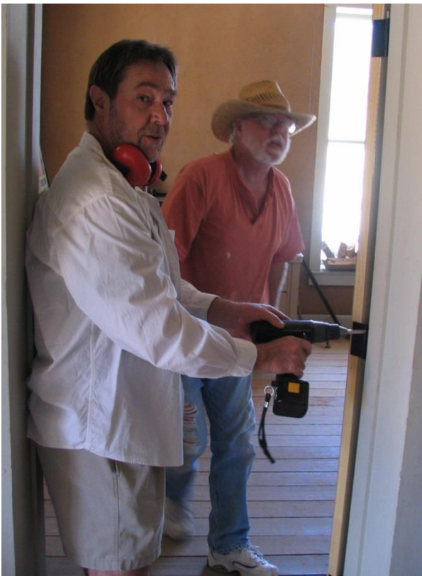
Photo courtesy of Mark Doumas John Weiss and Drum Haverstock install a door in the Headquarters Building at the 2007 work week.
