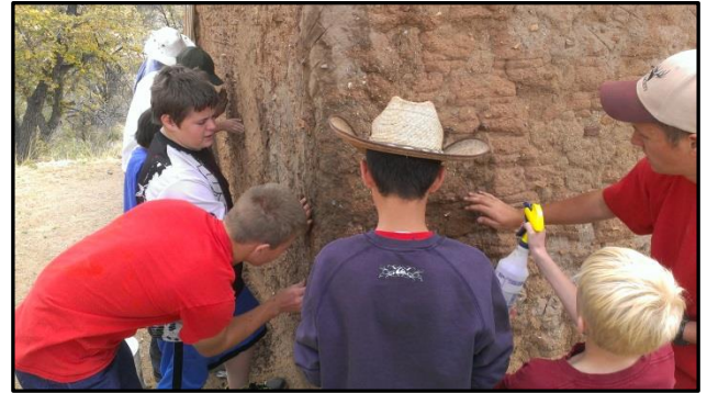
Scouts applying adobe mud to Gold Processing Building
