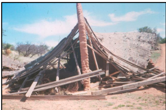
1992 - with collapsed roof
