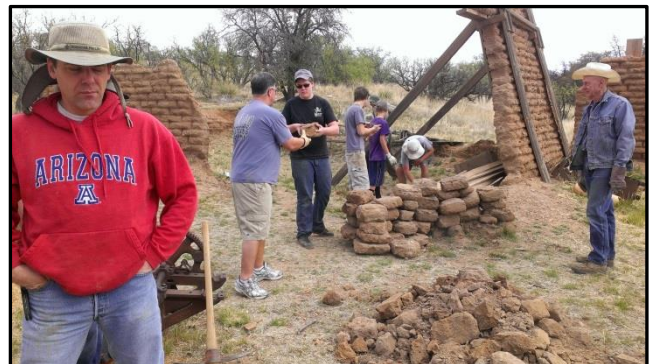
Retrieving fallen adobe bricks from the barn. Note the leaning barn wall
