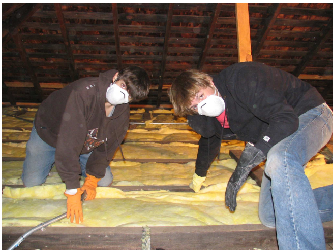
Max Schrager and Alex Doumas install insulation in the attic of the Headquarters building
