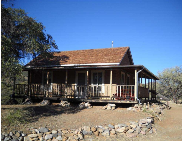
New Roof on Cabin C
