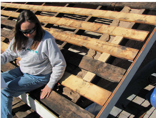
Kathy Makansi installs "mouse-prevention" blocking on the sub-roof of the rental cabin
