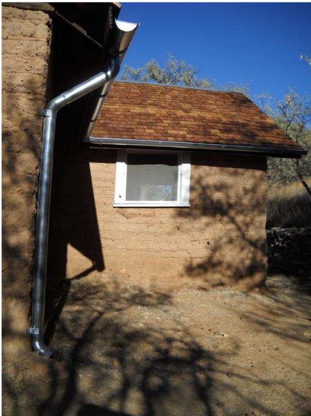
New roof and downspout on Cabin A
