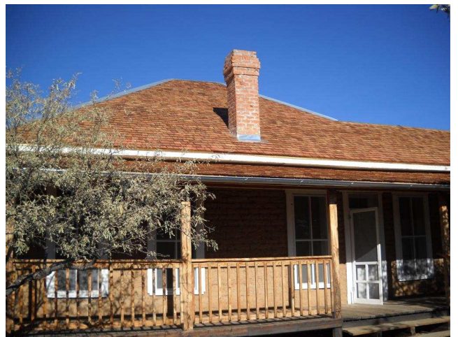
New Roof on Headquarters Building
