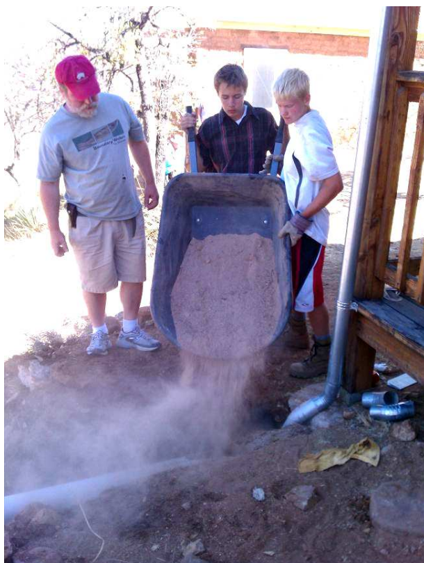
Scouts filling drainage-ways with soft sand
