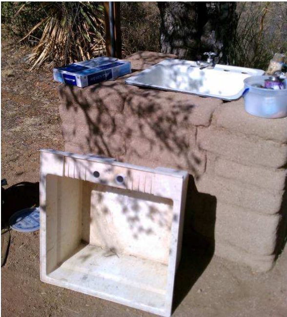
The old plastic sink outside the Headquarters Building has taken a beating from many years in the Arizona sun. A donated cast-iron/porcelain replacement has been installed.
