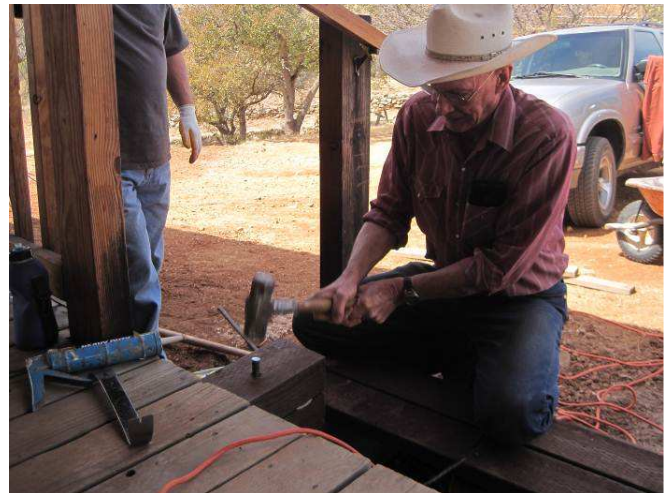
Pete Van Cleve rebuilds the front steps on the Headquarters Building.
