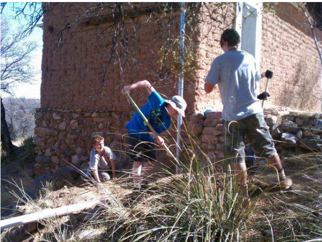
Scouts installing a downspout drainage pipe on the north corner of the Gold Processing Building
