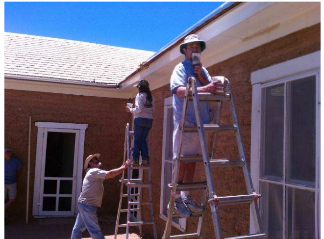
Chris Schrager, Kathy Makansi and John Weiss reposition gutters to better catch the rain.
