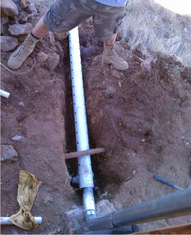
Some creative drainage pipe routing was required in order to dodge some buried historic plumbing.
