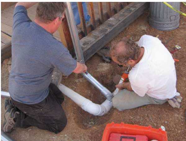
Steve and Chris connect a downspout to a drainage pipe.
