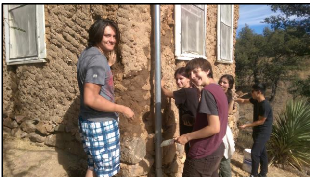
Verde Valley School students applying sacrificial mud coat to the exterior of the Gold Processing Building. Photo courtesy of Mark Doumas
