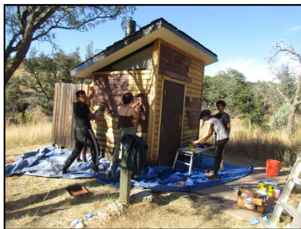
Both vault toilets had clap boards repaired and were painted. Photo courtesy of Chris Schrager
