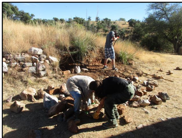
Verde Valley School students and staff repaired several slumping sections of retaining wall. Photo courtesy of Chris Schrager
