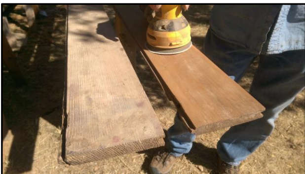
Rehabilitating floor boards from the Gold Processing Building. Left: Old and dusty. Right: clean, shiny and ready for another century of use. Photo courtesy of Mark Doumas
