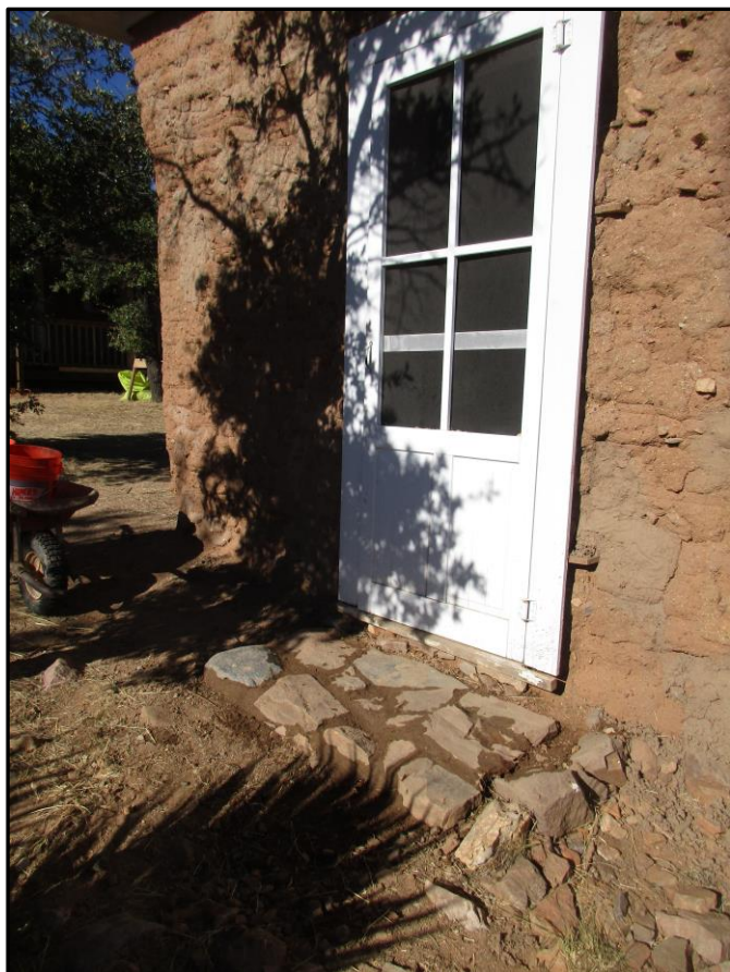
A new masonry landing for the main entrance of the Gold Processing Building. Photo courtesy of Chris Schrager
