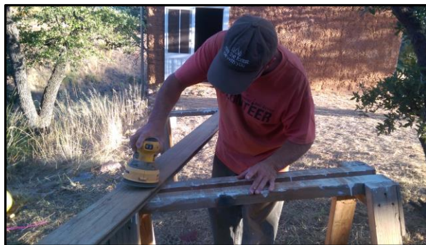
Doug Maus sands floorboards before reinstalling them in the Gold Processing Building. Photo courtesy of Mark Doumas
