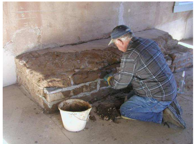
Jim Britton replaces adobe bricks on the Gold Processing "bench"
