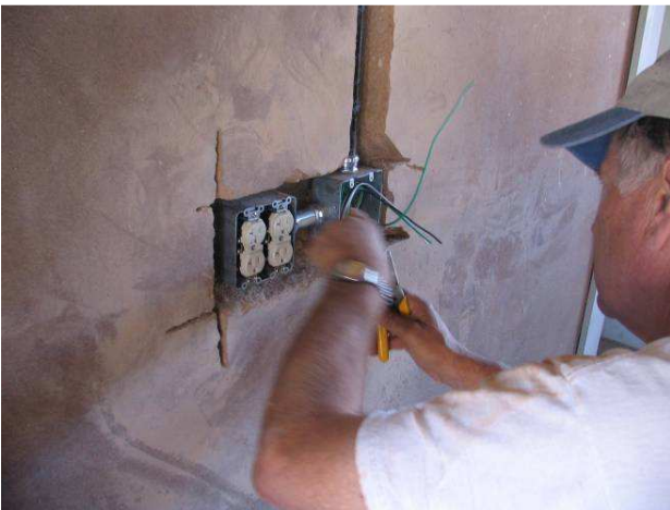
David Enge wires new outlets in Cabin C kitchen
