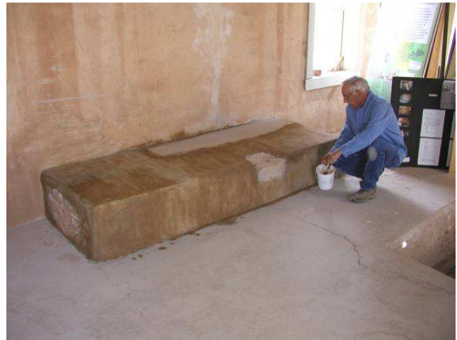
“After” - Jim Britton puts finishing touches on furnace bench
