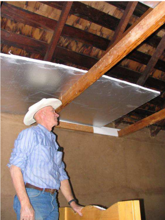
Pete Van Cleve re-installs ceiling insulation in Cabin C
