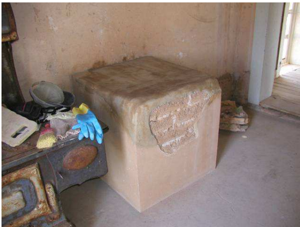
Gold processing building pedestal after restoration
