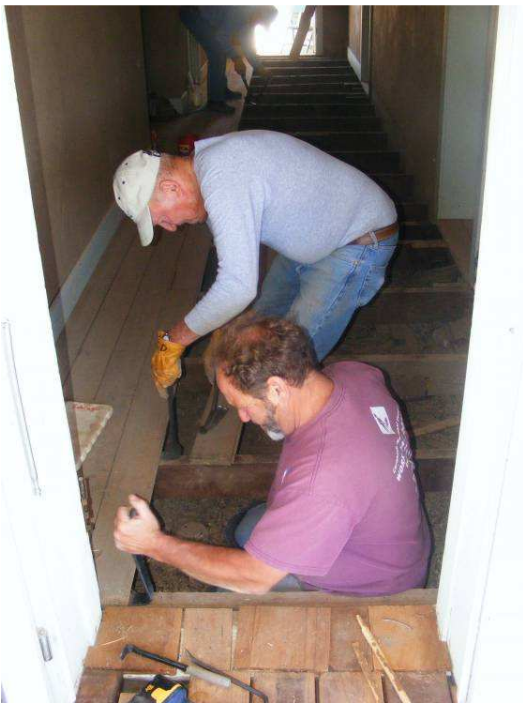
Chris Schragger and Ed Buell re-install floor boards
