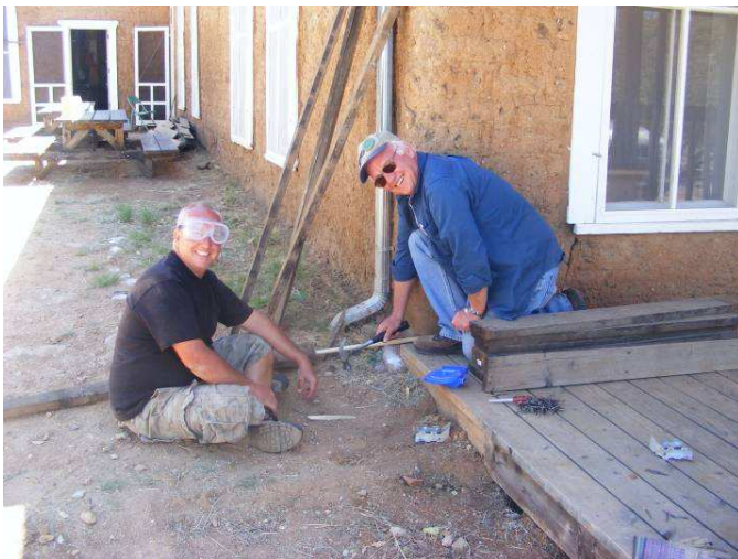
Doug Maus and Paul Batty rebuild ramp to the Headquarters building porch
