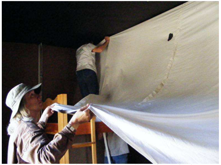
Mary Farrell and Kathy Makansi install newly washed manta ceiling in Cabin C
