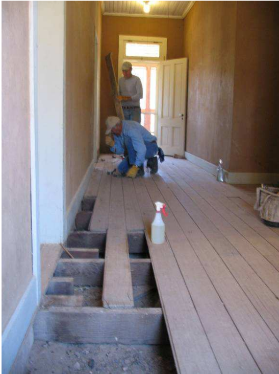
Jerry Mead and Ed Buell begin removing old Headquarters floor
