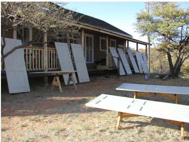
Freshly painted doors waiting to be re-installed in Headquarters building
