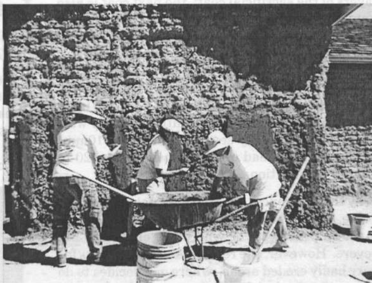
Applying the sacrificial coat.
