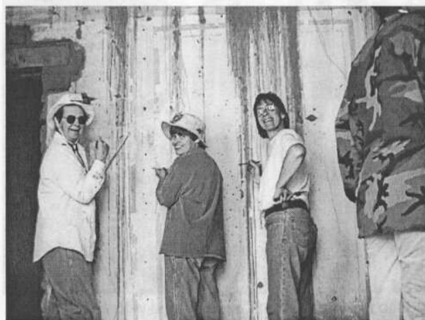
Verla Peter, Susan Jones, and KC Whiteley cleaning eroded mud off the painted surface.
