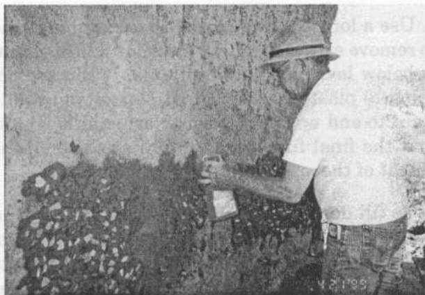
Note the small stones set in the wet mud to anchor the next layer.
