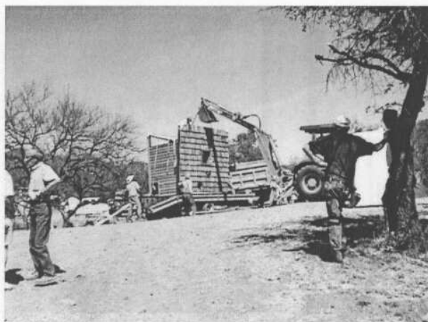
3. Backhoe prepares to set structure on pad.
