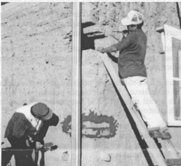
Jesus Robles and Jesus Romero add new bricks to re-bond walls of cabin at eroded corner.
