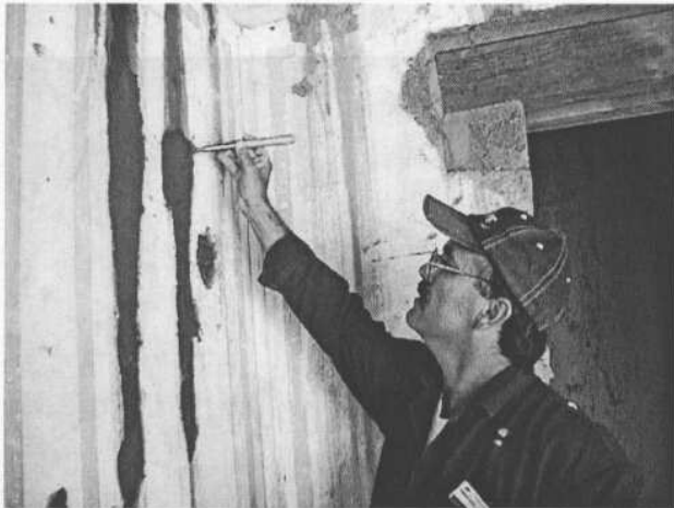
Rodolfo del Castillo using a tool tipped with an agate polishing stone to burnish edges of patch.
