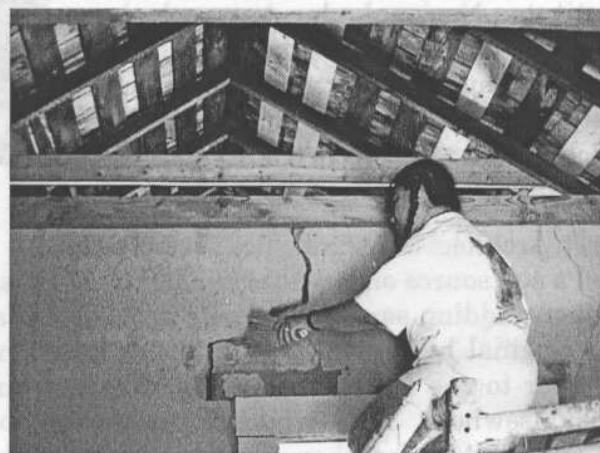
Martha Robles preparing crack for repair.
