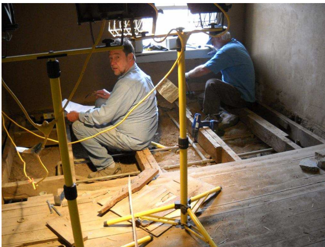
John and Drum record the plumbing underneath the bath room floor
