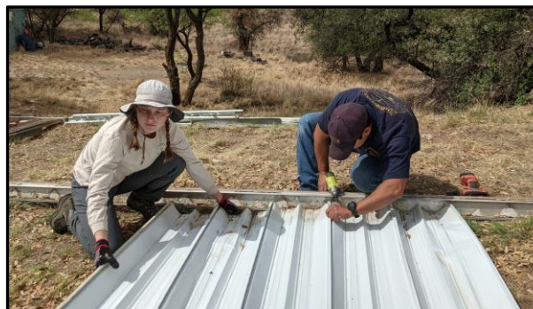
Disassembling the old aluminum trailer porch roof.
