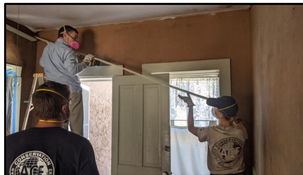
Removing the old manta
