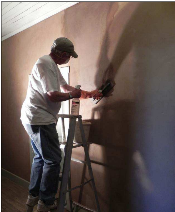
Jim Britton applies mud plaster to Headquarters Building hallway
