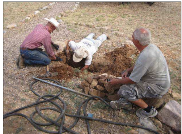
Pete Van Cleve, Chris Schrager and Doug Maus repair water line near rental cabin
