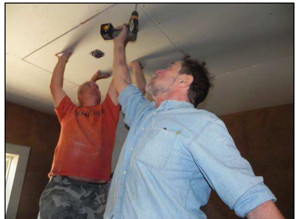
Doug Maus and John Weiss install drywall ceiling in rental cabin
