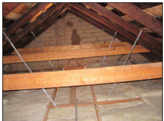
New ceiling joists, hangars and insulation were also installed
