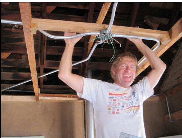
Mark Doumas installs new electrical outlets in rental cabin attic
