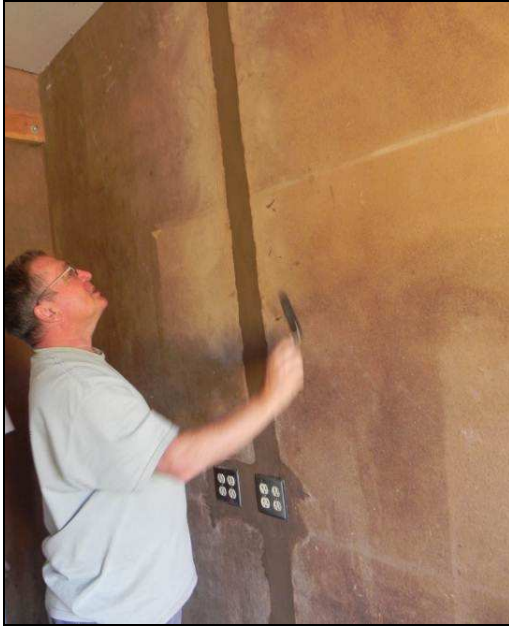
Steve Waylett plasters-over electrical conduit channels
