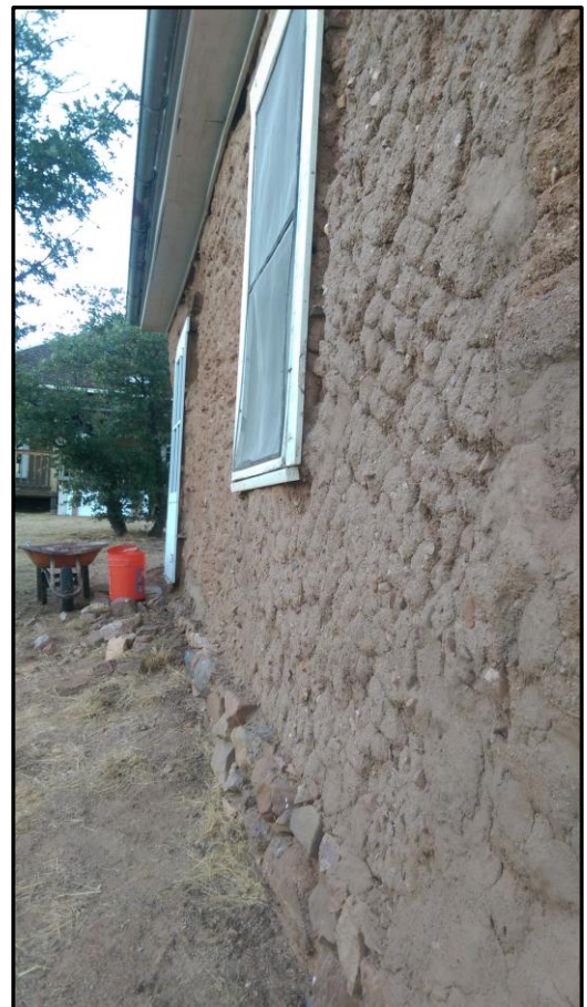
One of numerous adobe walls in need of new coating. Photo courtesy of Mark Doumas
