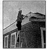
of fascia board behind the gutter. Turns out, the entire fascia strip under the gutter was riddled with carpenter bee tunnels. The entire gutter and fascia strip were removed. A new fascia board was installed and we have a new gutter to be installed at a future work day.
