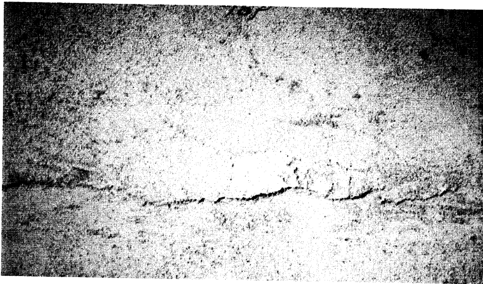
Figure 14 - This is a close up of the "plaster line" that appears between each of the four 2 x 4 gringo boards along the west wall of Room E-2. The overlap of the plaster indicates that the area below the 2 x 4s was applied last.
