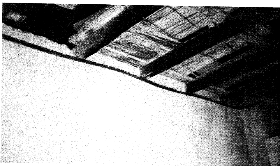
Figure 4 - This shows the north wall of Room E-1 with the wood trim nailed to the bottom of the ceiling joist. This trim board was along all four walls and had been used to hold the manta cloth in place.
